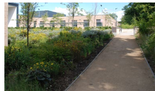
Recently surfaced routes at the New REH Building; wide, smooth, permeable surfacing which is inclusive and attractive within its woodland setting.
